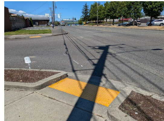
Curb ramps misaligned at S 40 th St
