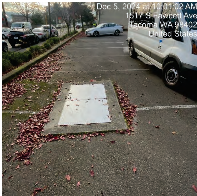
Figure 2: Top photo of oil water separator in parking lot.
